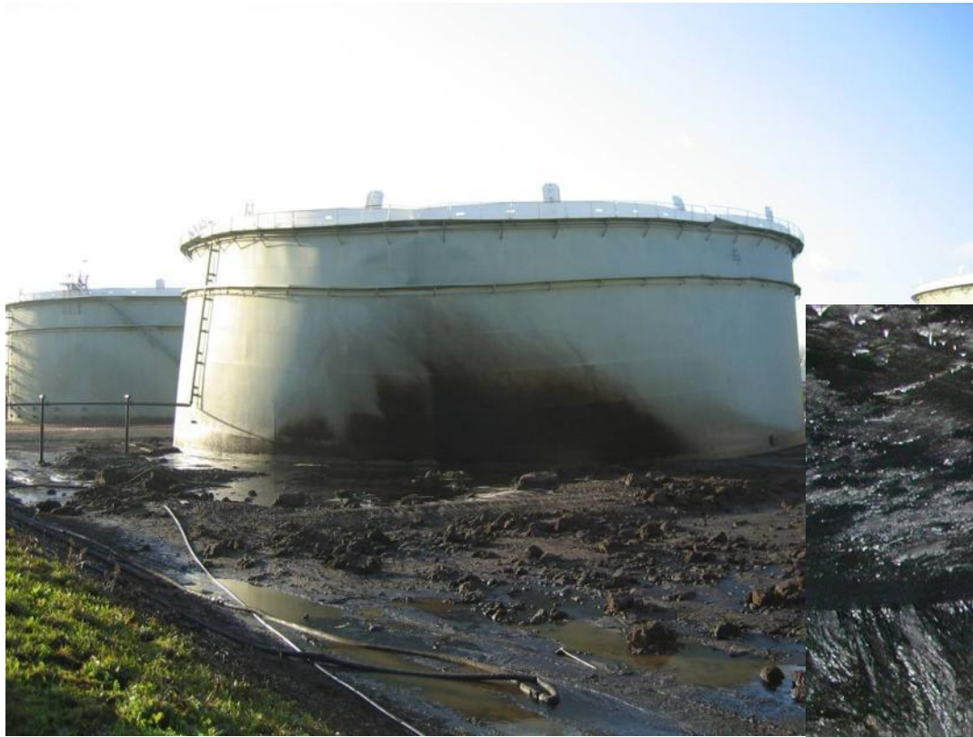
Internal corrosion of an oil tank
