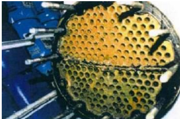
Heat exchanger tubes in Cu-Ni 90-10
